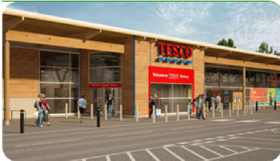
It's made from timber, uses sun-pipe lighting and collects rainwater to flush the toilets and run the car wash.
